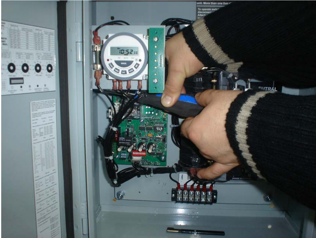
Figure 2. REMOVING THE TIMER SUPPORT BRACKET
